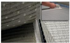
6 Apply another layer of C2 / S1 tile adhesive on the cured composite sealing using a spreader comb with 1/4" teeth.
