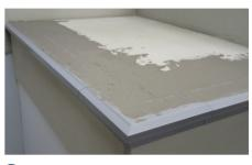
Apply filler to level out any difference in height of the floor between the profile and the screed.
