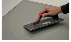
**8** Grout the tiles after the specified curing time of the tile adhesive used has elapsed. Use a flexible grout to EN 13888 CG2 and process according to the manufacturer's instructions.
