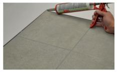
Oreate expansion joints in the tile surface in line with applicable codes of practice. Take format sizes and the location of the surface into consideration during planning. Seal expansion and connecting joints with a permanently elastic, neutral curing silicone sealant.
