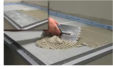
Z Lay the tiled surface after the curing time of the thin bed mortar has elapsed. Lay the tiles in a thin bed of flexible adhesive mortar suitable for outdoor areas.
