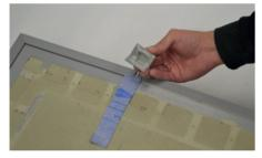
4 Glue the profile joints up to the groove with BLANKE AQUA SHIELD and AQUA SEAL. Then affix the BLANKE Balcony Gutter Edge Protector joiner with BLANKE AQUA SEAL.
