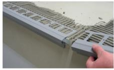
Spread tile adhesive C2 / S1 at the edges, fit joiners in the joints of the BLANKE Balcony Gutter Edge Protector Profiles and
