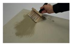
All substrates must be capable of bearing the load and free of any layers that could impair bonding. The substrate must comply with level tolerances to ANSI A-108.01-2.6.2 and have a slope of approx. 1.5-2%. Apply a primer coating suitable for the substrate and its surface condition. Observe manufacturer's specified drying time.
