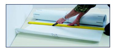
**5.** Cuts can be easily made using a knife or a scissors.
