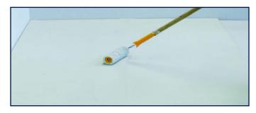
**1.** Substrate must be solid, flat, load-bearing and free from bond-inhibitors. Any loose material must be ground off. Primers for moisture sensitive substrate and self-levellers should be applied as needed.
