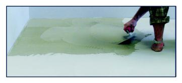
**2.** Using a utility knife, dry cut the mat to fi the area where the tile will be installed. Be sure to allow a minimum of 1/4" gap where the installation meets vertical surfaces, thresholds and different floor types. Apply a normal mix of latex-modified thinset mortar (midgrade quality or higher) to the substrate with a 5/16" V-notched trowel
