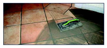
**7.** Grout the tile after allowing the curing period as recommended by the grout manufacturer. Follow the manufacturer installation instructions and industry practices when grouting.
