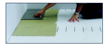
**6.** Allow the thinset to set-up until hard. Traffic on the BLANKE SECUMAT should be kept to a minimum while the thinset is curing. Apply latex modified thinset (midgrade quality or higher) and install tile following the thinset manufacturer installation instructions and in accordance with industry practices in the same way as tile is in-stalled on backerboard and similar underlayments.
