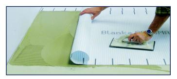
**4.** Butt the edges of adjacent sections tightly together.
