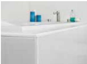
Outside wall edge protection
