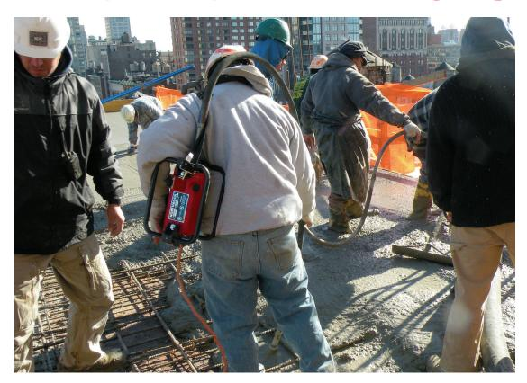
The Northrock Pro Series of electric vibrators includes three models that range from the Pro 1.5 for small jobs requiring a 1 1/2" head or less, to the Pro 2 + the most versatile motor on the market that can power up to a 2 1/2" head, and finally the Pro 3 which is a true work horse for the most demanding applications.
