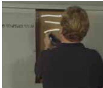
Apply silicone to backing
