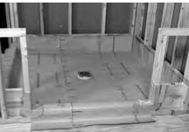
Installed in a full mortar bed method shower with Chloraloy® shower pan liner and preformed Outside/Dam Corners.
