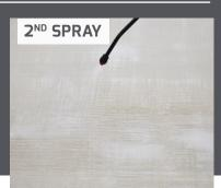
After first coat is dry to the touch (approximately 2-4 hours), apply an undiluted second coat in a light, even coat at a rate of approximately 160 ft²/gallon\*.
