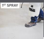
Using a handheld, airless type sprayer, apply first coat at a rate of approximately 60 ft²/gallon\*\* or until rejection.
