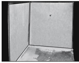
NOTE: Sections of HYDRO BAN® Sheet Membrane may also be shingled (overlapped) during installation without the need for HYDRO BAN Sheet Membrane Sealing Tape. The top section must overlap a minimum of 2" (5cm) onto the bottom section of HYDRO BAN Sheet Membrane.
