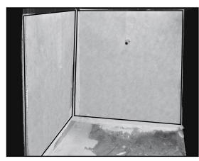
Best practice; sections of HYDRO BAN Sheet Membrane should be butt-jointed and the seam between the HYDRO BAN Sheet Membrane sections should be covered with HYDRO BAN Sheet Membrane Sealing Tape installed with the appropriate thin-set. Make sure that the HYDRO BAN Sheet Membrane Sealing Tape overlaps each HYDRO BAN Sheet Membrane section by a minimum of 2" (5 cm). The floor should be the last section installed.
