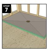
Apply thinset to the back of your shower pan using the smooth side of a trowel. Do not apply thinset on or within ½" of the stainless steel drain support ring.
