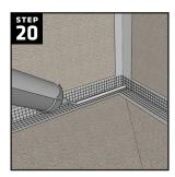
Apply a continuous ½" bead of joint sealant into the corner seam of the shower pan where it meets the curb or wallboard. Use the corner putty knife to smooth out the sealant so that there is at least 1" of sealant on either side of the seams.
