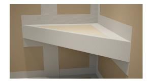
6. Apply a layer of thin-set and wrap the exposed sides and brackets in provided tape.
