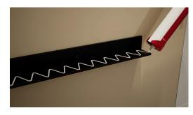
3 Apply adhesive to the brackets, and then set the bottom board onto the brackets.
