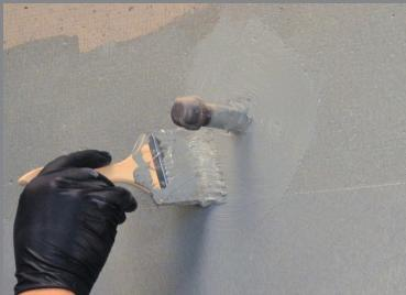
**Coverage Rates** 3.5 gal. (13 L) unit - 195.5 sq. ft. (18 sq. m) 2 coats over drywall
