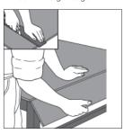
To make cutouts for pipes and fixtures, use a utility knife to cut through facers on both sides and remove foam core. Or, use an electric drill with a hole-saw bit.
