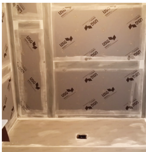
USG Simply apply sealant over fasteners
