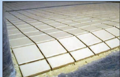
Handi-Kirb™ thin bed finished Acabado del Handi-Kirb™ delgado
