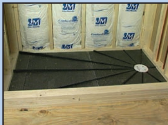
Pre-Pitch™ Standard and Extended installed in rough-in.
