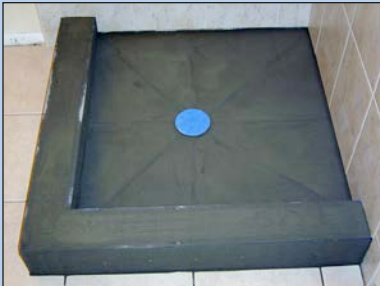
Kirb-Perfect® filled with mud Kirb-Perfect® relleno de mortero
