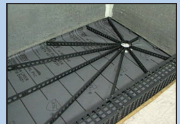
Quick-Pitch® Standard and Extended and Kirb-Perfect® installed.
