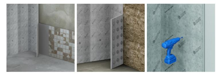
• <u>Assembly of the panels</u> used to create walls for shower cabins and furnishing elements may be carried out using a <u>hybrid</u> <u>sealant</u>, such as **Mapeflex MS45**, and mechanical fasteners.
