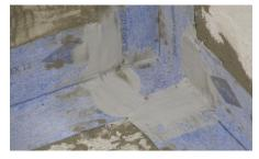
4 Flatten out any excess BLANKE AQUA SEAL at the connections of corners and bands as shown in the picture.
