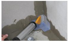
In applications subjected to constant and extremely moist conditions, use BLANKE AQUA SEAL waterproofing adhesive to seal the overlapped seams.
