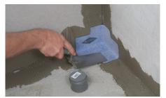
Treat drains, pipe surrounds, corners, wall-to-wall connections and wall-to-floor connections first. Here shown: Inside corner. Apply the thinset to the substrate by using 1/4" x 3/16" V-notched trowel. Press BLANKE AQUA CORN I into the thinset by using the flat side of the trowel, ensuring 100% contact with the substrate. Make sure to press out any air pockets.
