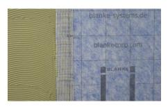
The edges of adjoining BLANKE AQUA SHIELD 100 sections have to overlap by at least 2 inches.
