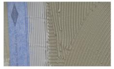
When installing sheets of BLANKE AQUA SHIELD membrane, use thinset on the wall or floor area and BLANKE AQUA SEAL on overlapping seams. Always overlap 2 inches to ensure watertight connections.
