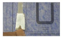
9 Again flatten out any excess BLANKE AQUA SEAL at the seams as shown in step 4.
