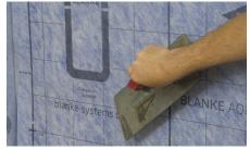
6 Use the flat side of the trowel to ensure 100% contact with the substrate. Make sure to press out any air pockets.
