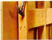
2. Expand bench to width desired, being sure to keep large holes in front face of BB-ADJR aligned for both halves. Secure final dimension as detailed in placement instructions, **Step A and C.** *Step B, "Face stiffener" is not required with INVISABOLT system.*
