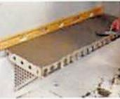
5. Tile and grout the top, face and exposed sides of BB-ADJR and BT-17S as desired.
