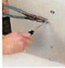
3. Inject a small amount of caulk in each mounting hole and re-position BB-ADJR. Install all screws and secure BT-17S to BB-ADJR. Add additional caulk over screw heads and a continuous bead along top edge of bench where it abuts wall.
